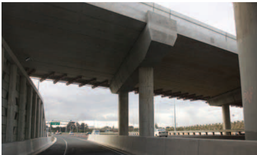
North Shore's new Esmonde Road interchange improves motorway access and allows drivers, cyclists and pedestrians to move freely across the highway between Takapuna and Northcote.
